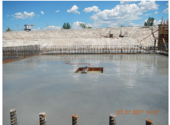
Figure 2 – Completed Digester Floor; Sprinkler Keeping Slab Wet
