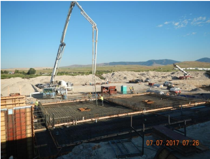
Figure 1 – Digester Floors Concrete Placement
