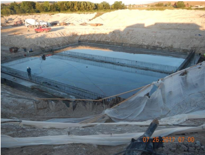
Figure 3 – SBR Basin – Foundation Completed, Covered with Water for Curing
