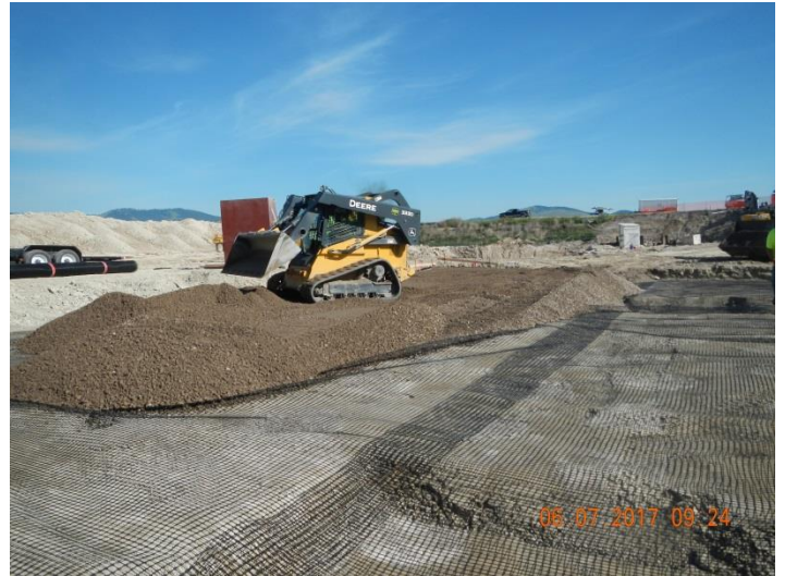
Figure 2 – Foundation Reinforcement Fabric Under Digesters
