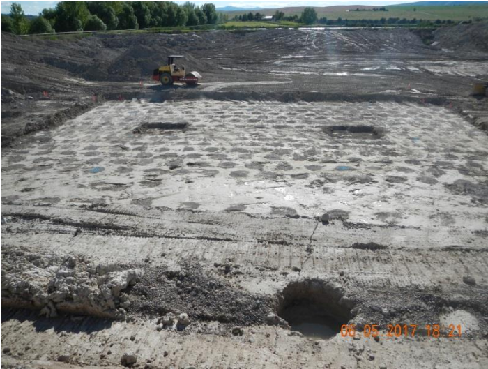
Figure 1 – Digesters: Completed Engineered Aggregate Pier Installation
