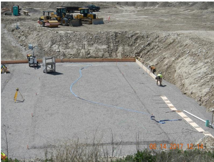
Figure 3 – SBR Basin – Foundation Preparation
