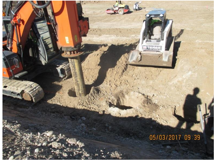
Figure 2 - Engineered Aggregate Pier Installation
