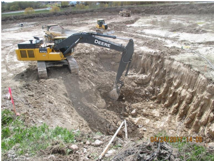
Figure 3 - SBR Basin Excavation
