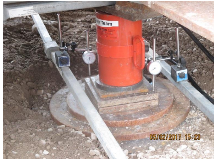
Figure 4 - Required Load Testing of Pier
