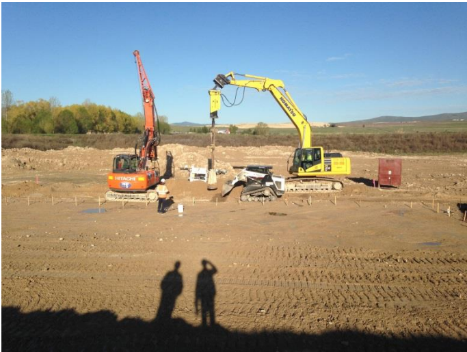
Figure 1 - Engineered Aggregate Pier Installation
