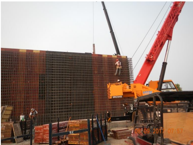
Figure 3 – Rebar Typing in North Digester Tank Wall
