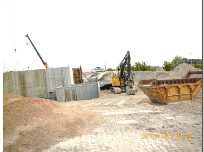
Figure 2 – Completed Digester South Wall; Polymer Feed Equipment Room
