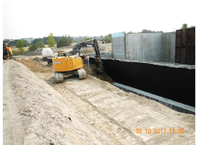
Figure 4 – Backfilling on East Side of Control Building Basement
