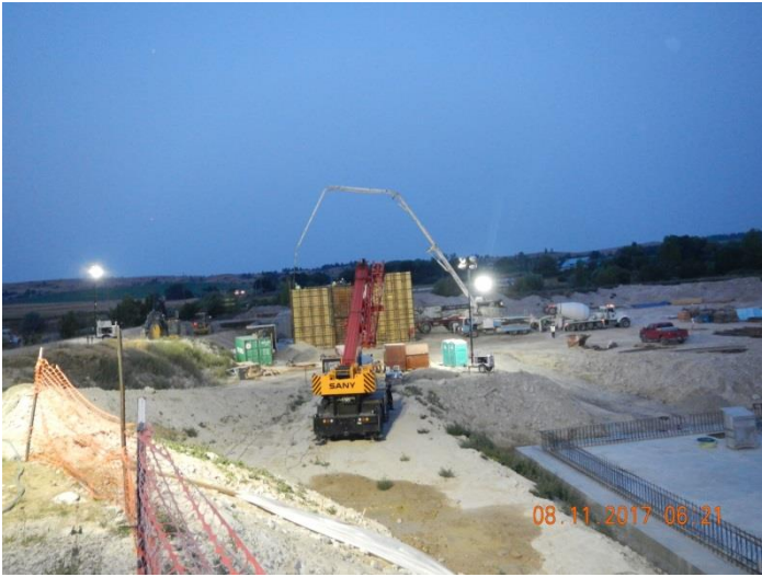
Figure 1 – Early Morning Concrete Pour – Digester Walls
