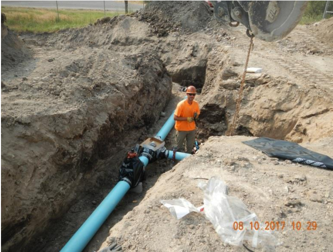
Figure 5 – New Potable Water Main Across Kerr Dam Road to New Plant
