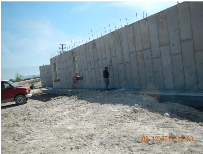
Figure 3 – Headworks Building Basement, West Side
