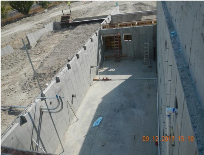
Figure 1 – Control Building Basement
