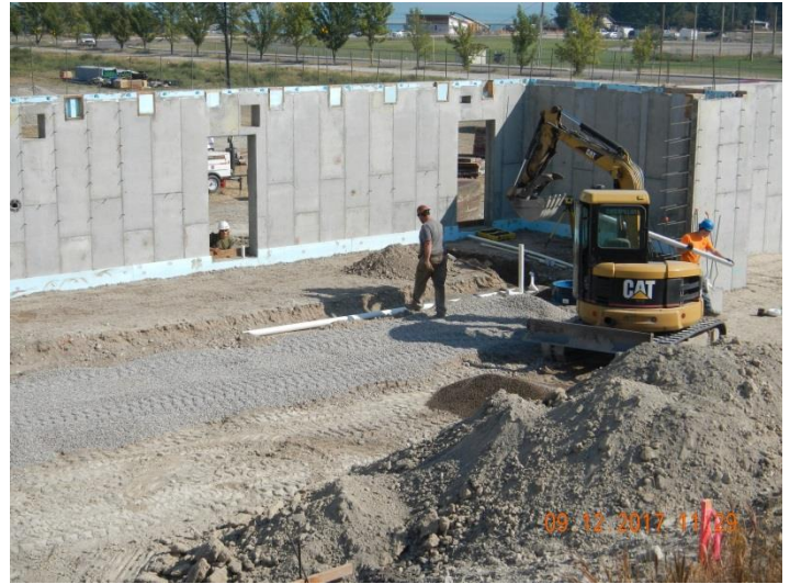
Figure 2 – Headworks Building Basement
