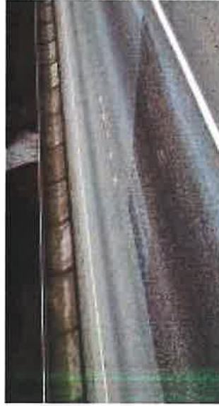
Chip Seal Repair Low
