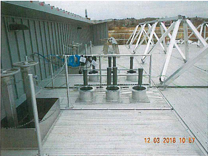
Figure 9 - Instrumentation Install; Digesters
