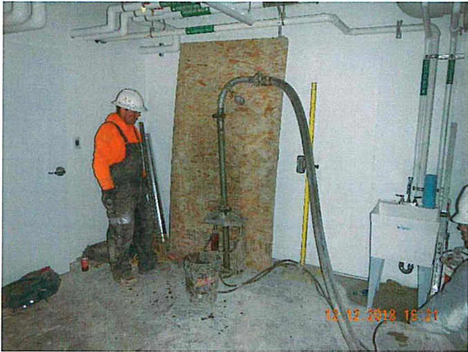
Figure 3 - Compaction Grouting: Basement of Headworks Bldg.
