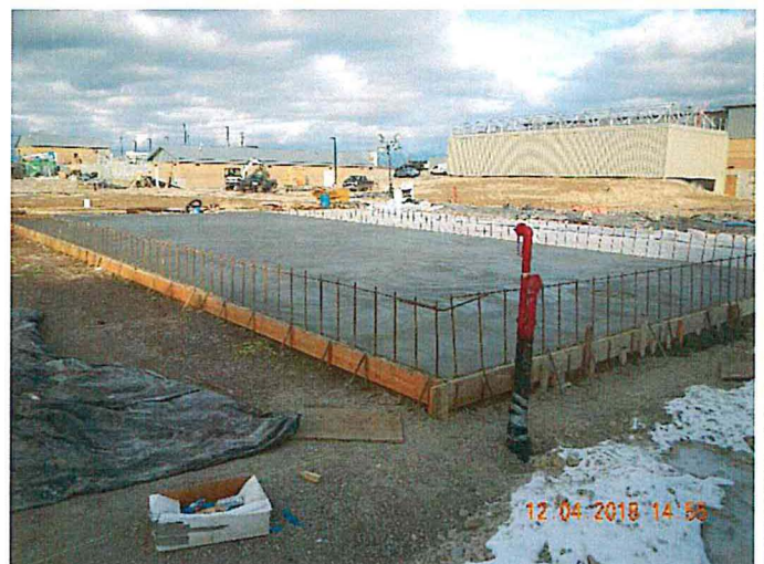
Figure 12 - Sludge Drying Beds - Completed Slab #2
