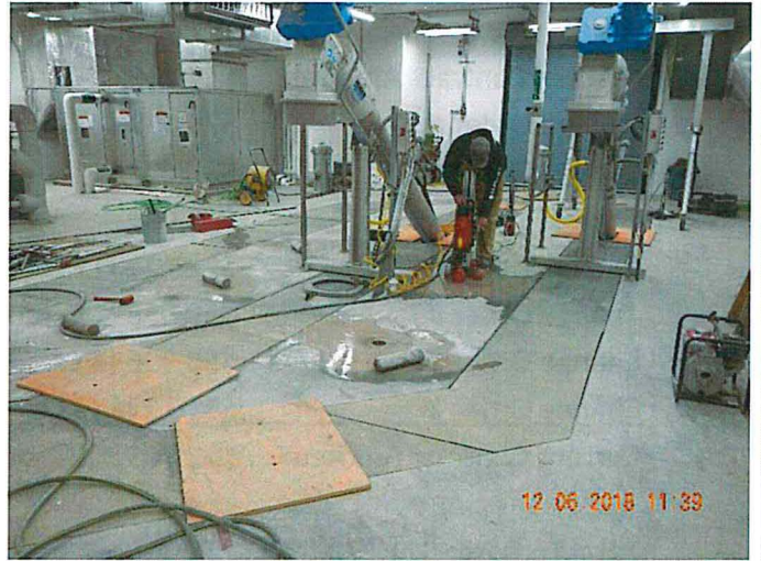
Figure 4 - Coring Concrete for Compaction Grouting; Upstairs Headworks Bldg.
