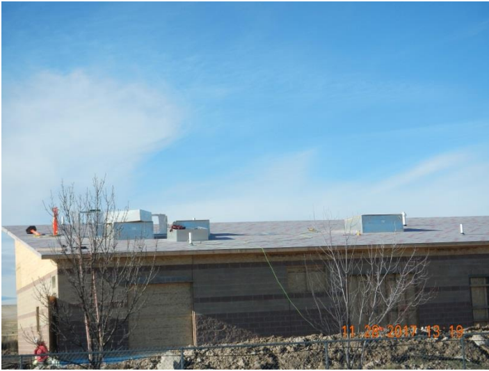
Figure 7 – Control Building Roof and HVAC Equipment Provisions
