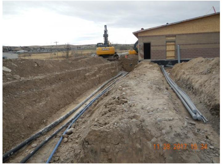
Figure 8 – Water Lines & Electrical Conduit Runs
