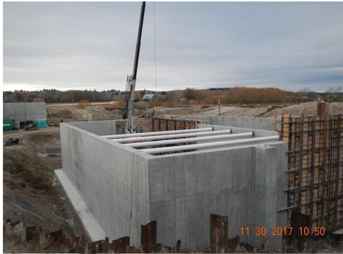
Figure 3 – SBR Tanks – Center Wall Pour (1 of 2)
