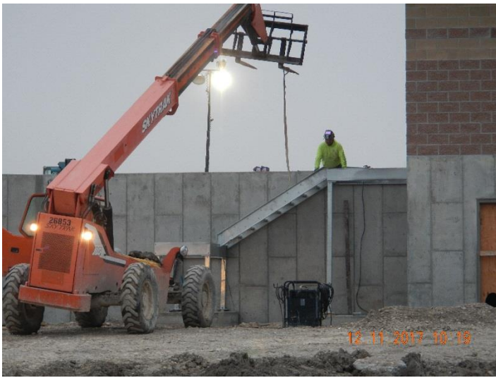
Figure 1 - Headworks Bldg. Ext. Stairs
