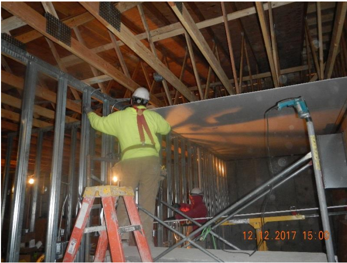
Figure 7 - Control Building - Upper Floor Framing and Drywall
