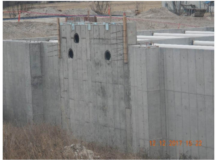
Figure 2 - North Wall of SBR - Complete
