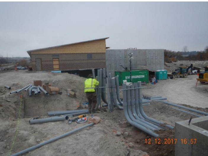
Figure 5 - Electrical Site Work
