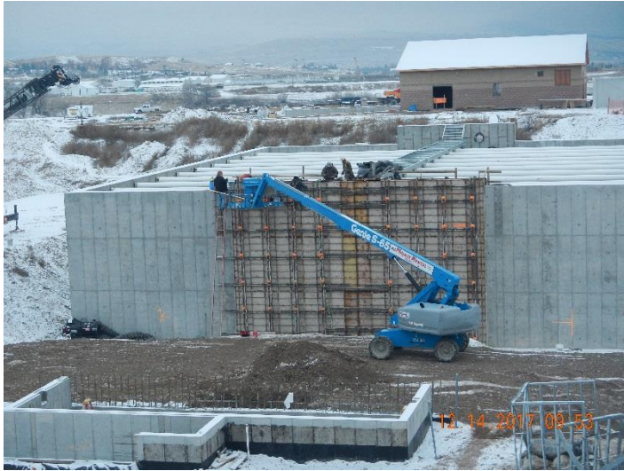
Figure 3 - South Wall of SBR- Last Pour
