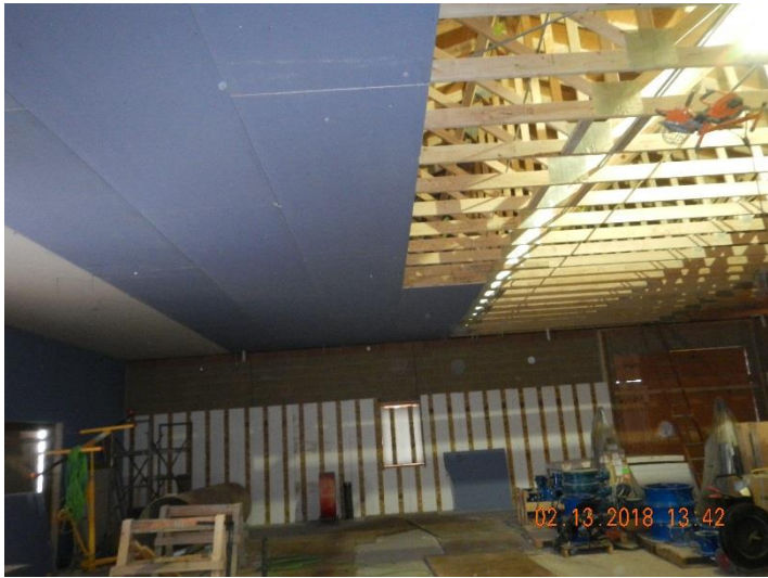
Figure 2 - Headworks Bldg. Interior Wall Insulation
