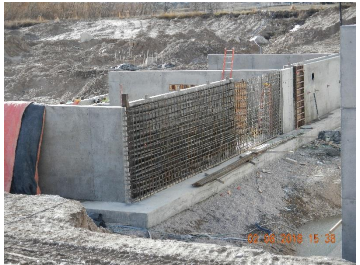
Figure 3 - Post EQ Basin North East Wall - Forming
