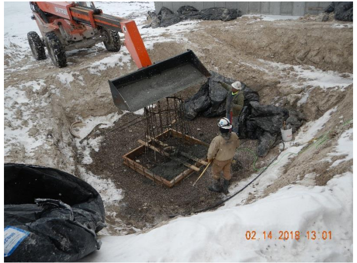
Figure 1 - Grit Chamber Base - Form Work
