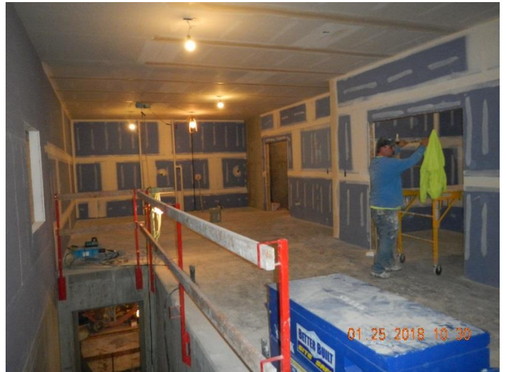
Figure 6 - Control Building - Dry Wall; Chem Feed Area
