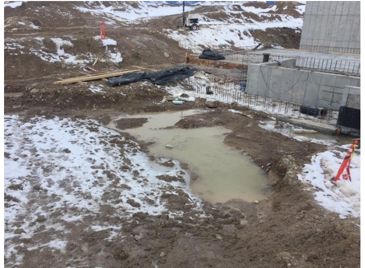
Figure 8 - Wet Site Conditions
