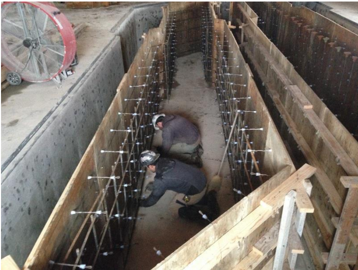
Figure 1 - Headworks Flow Channel - Forming
