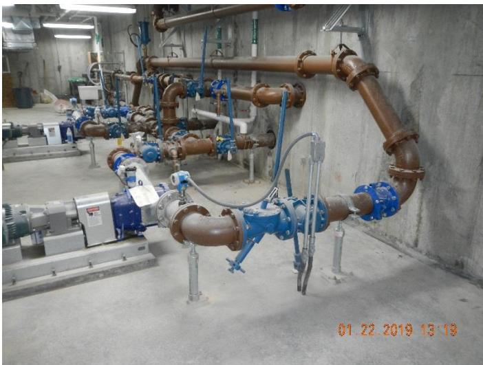
Figure 3 – Control Building Basement. Digester Leaks Repair Progress
