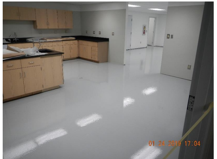
Figure 4 – Control Building Lab/Office, Floor Coating
