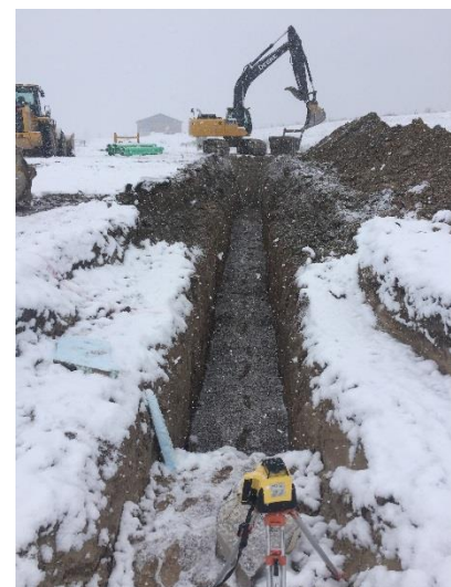
Figure 6 – Storm Pipe Installation
