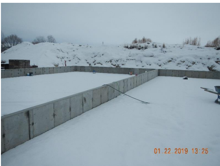
Figure 5 – Sludge Drying Basins #1/#2 Perimeter Walls
