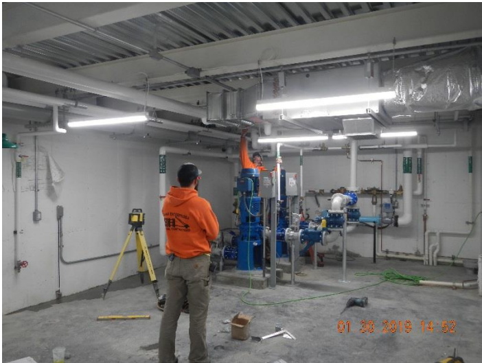
Figure 1 - Installing Grit Pump Hoist Rail in Headworks Basement
