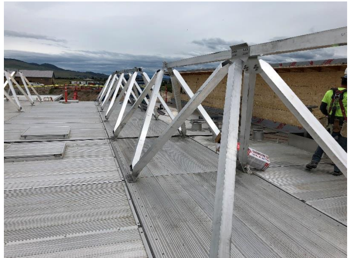
Figure 10 - Digester Roof Structure; Completed
