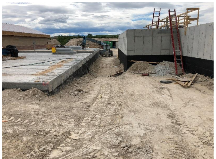
Figure 6 - SBR Outlet Vault, Completed Walls
