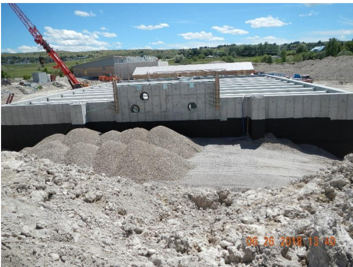
Figure 5 - SBR Inlet Vault; Backfill
