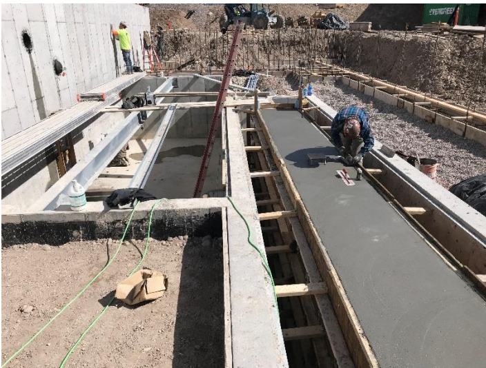
Figure 3 - UV Disinfection Channel Completion
