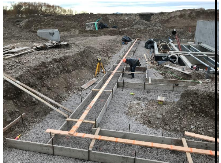
Figure 4 - UV Building Wall Footing Forms
