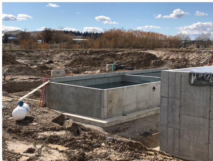
Figure 5 - Completed Post EQ Tank; Leak Testing
