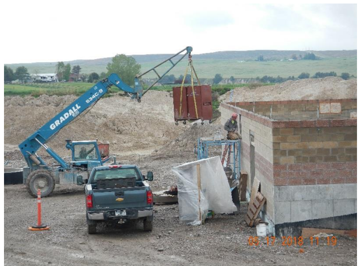
Figure 6 - UV Disinfection Building - Masonry
