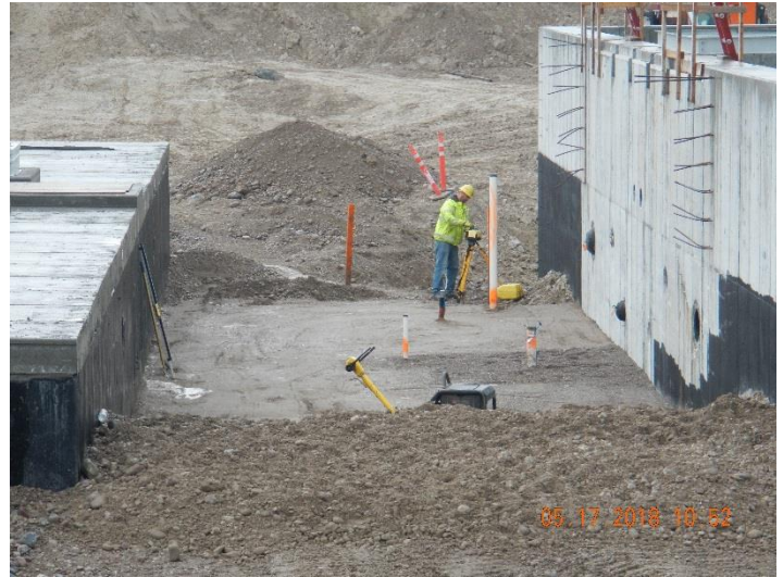
Figure 4 - SBR Outlet Vault Preparation
