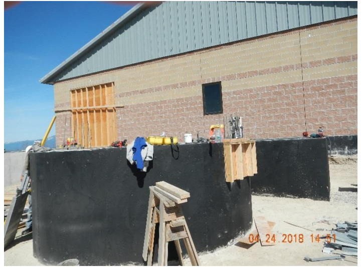
Figure 2 - Upper Grit Chamber Walls
