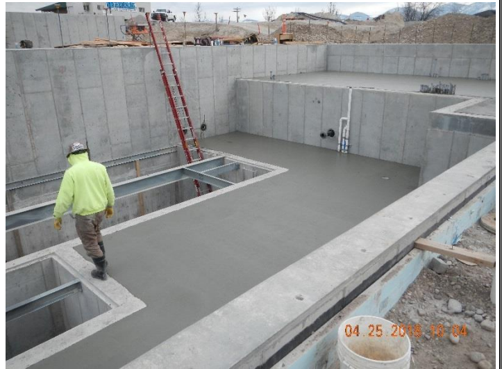
Figure 4 - UV Building, Finished Floors
