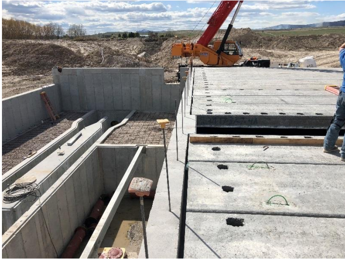
Figure5 - Roof Over Post EQ Tank, UV Channels
