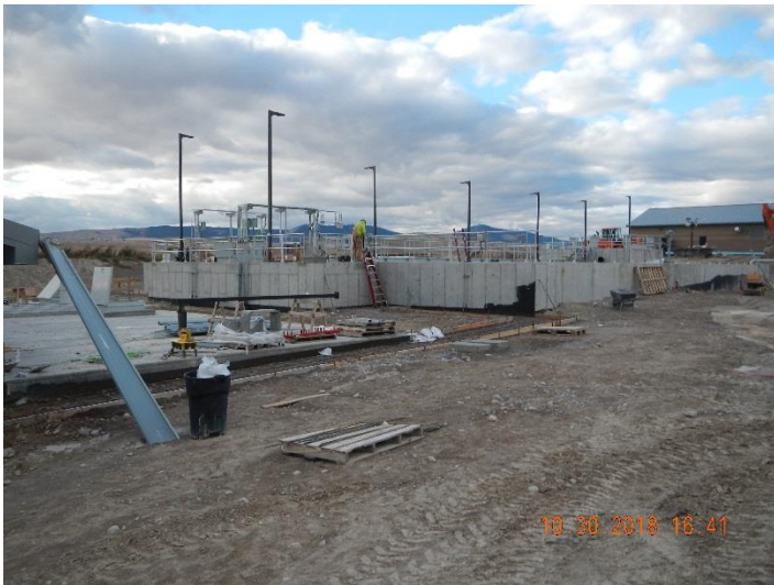
Figure 1 - SBR Final Grading, Lighting, Electrical
