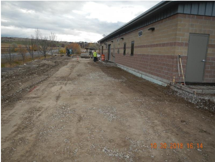
Figure 6 - East Access Road, Sidewalk Prep.
