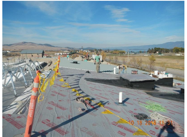
Figure 2 - Control Building Roof In Process
