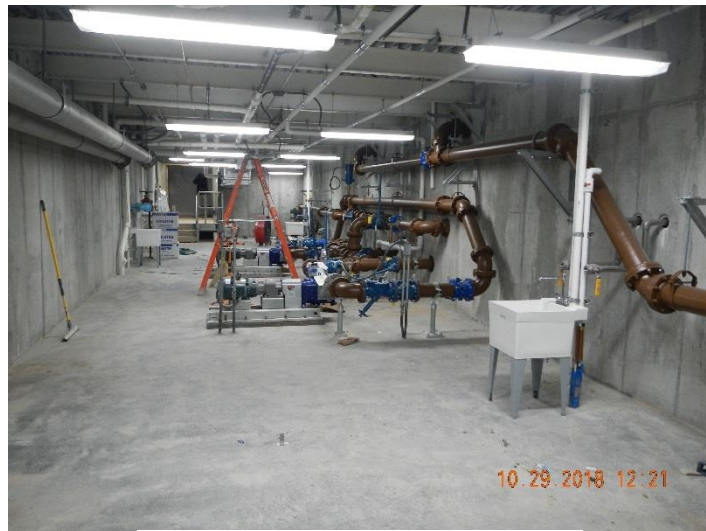
Figure 1 - Control Building Basement (Dry)
