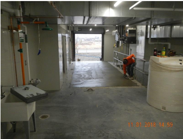
Figure 3 - Control Building Floor Repair, Complete
