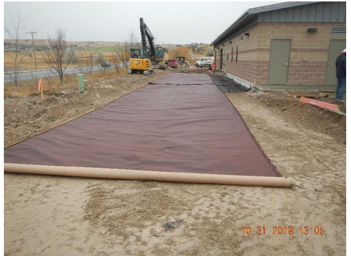
Figure 7 - East Access Road, Geocomposite Placement
