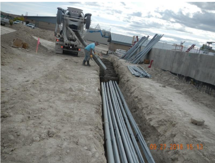
Figure 5 - Electrical Duct Banks; Concrete Encased
