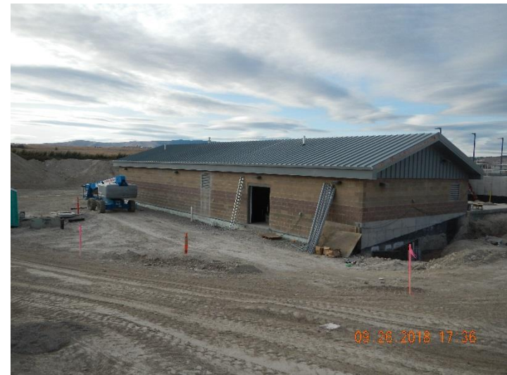
Figure 6 - UV Building - Roof Complete
